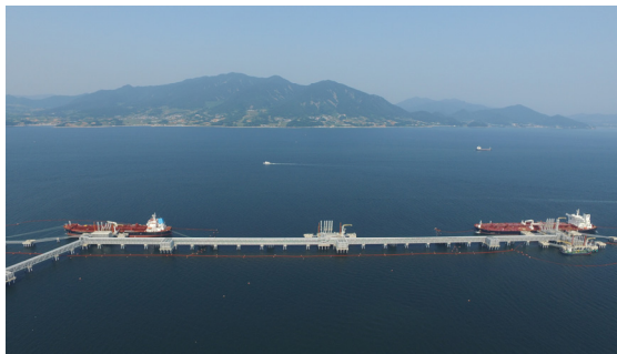
(a) Overview of tank terminal
