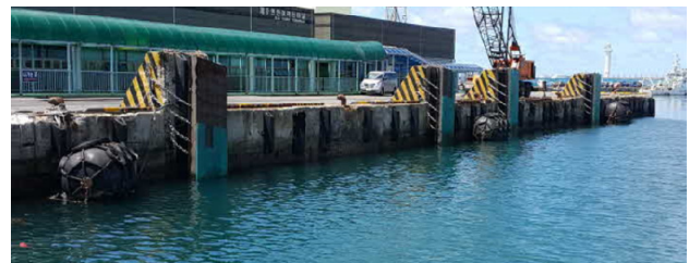
Fig. 2. Status of fender for No.24 berth
