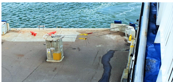
Fig. 9. High height bitt of west harbor terminal in Helsinki
